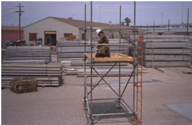
Attach a ladder for access to the second level. Install the guardrails, midrails, and toeboards. Secure the steel plates/gratings to the bearer.
