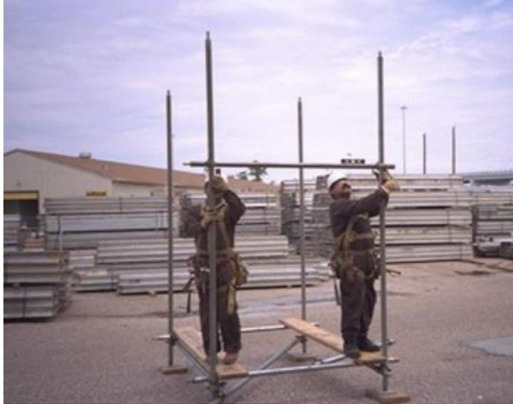
After ensuring the first level is properly spaced, square, plumb, and level, you may begin the second level. It is best to have the clamp spacing preset on the horizontal tubes by measuring the spacing with a tape measure. Do not exceed 6'6" to this second level.
