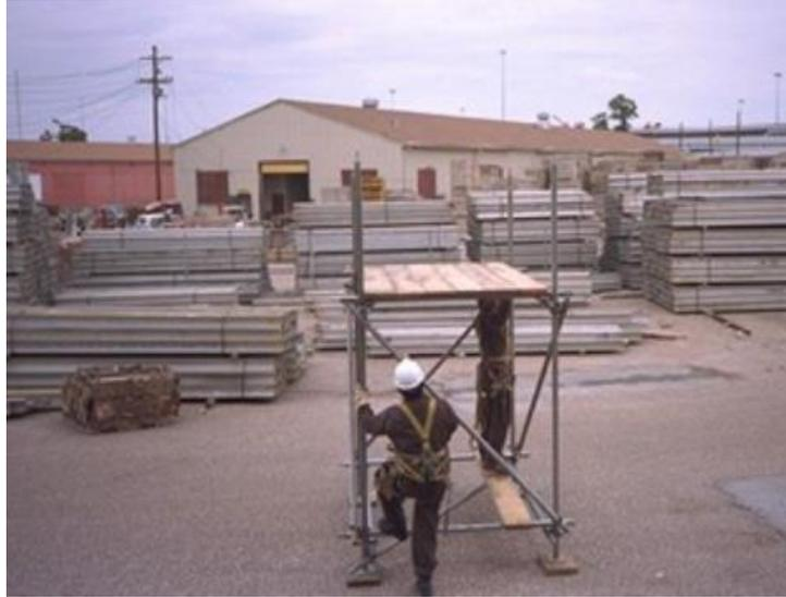
Put the steel plates/gratings for the second level on the bearers. Once the erector climbs to the second level, he will be exposed to a fall hazard and precautions to be taken
