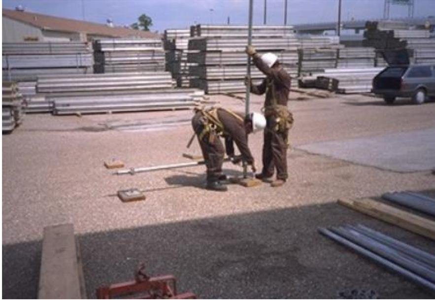
Lay out the mudsills at approximate centers and place base plates on them. The bearer is the name for the tube goes across the scaffold that the boards rest on. The runner goes down the length of the scaffold. Lay these out and stand up the first post. Clamp the runner to the post close to the base. Clamp the bearer on at 90 degrees on top of the runner.
