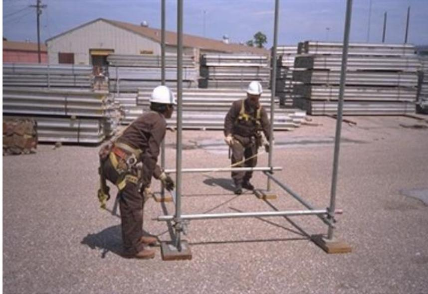
After all four posts are attached, measure the scaffold from inside to inside to insure the corner angles are at 90 degrees (square).
