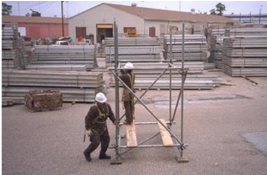
Attach the second level bearers and runners. Next, attach the diagonals. Swivel clamps are used to attach these at an approximate 45 degree angle from level to level. All four sides should have diagonal bracing attached.
