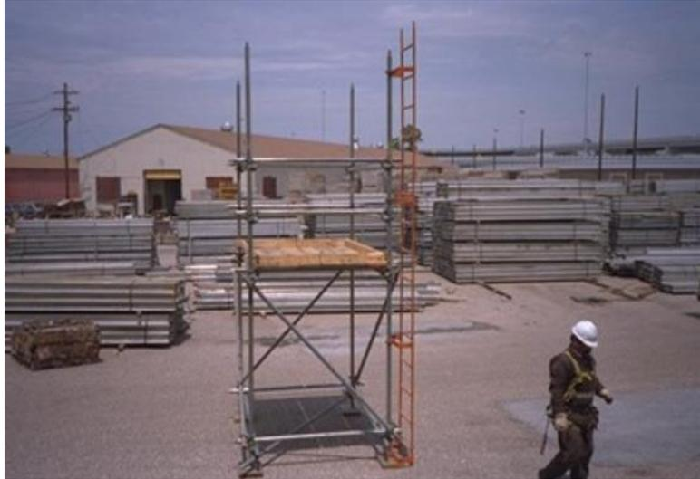
The completed scaffold should be square, rigid, properly diagonally braced, ladders should extend at least to top of handrails, work platforms fully covered with steel plates/gratings, toeboards installed, screening attached where required, guardrails & midrails installed, and all other safety measures met.
