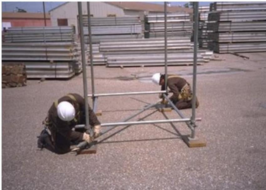
It is a good idea to attach a horizontal diagonal at this time to ensure that the scaffold remains square. Make sure the legs are level and plumb as you go.
