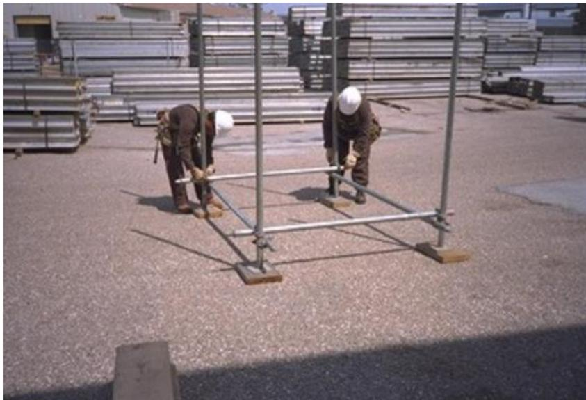
After the first post is upright and runner and bearer attached, the scaffold will be self supporting. Next, attach the other posts at predetermined centers. The bearer always goes on top of the runner for a safety clamp backup effect.
